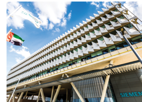
Siemens Middle East HQ at Masdar City
