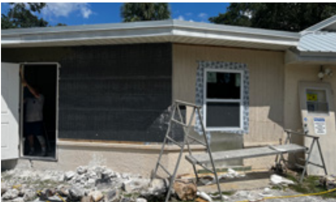
The old door opening is sealed off.
