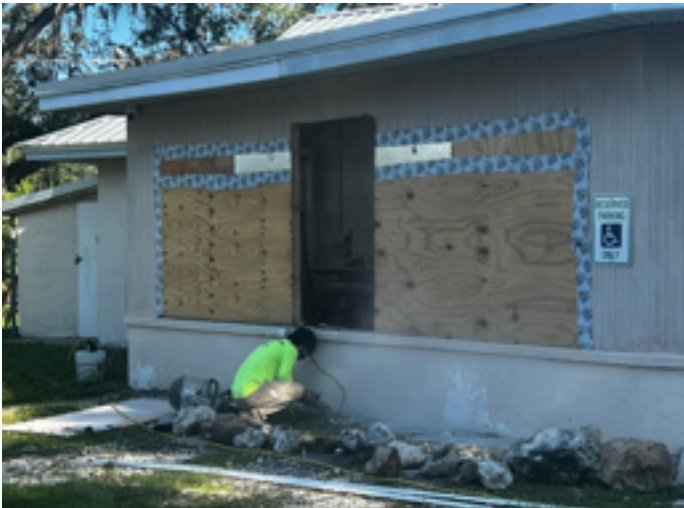
Cutting open a new opening for the door.
