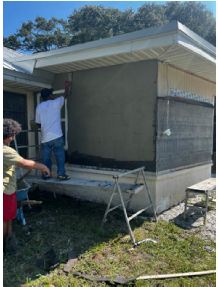
Finishing the outside with stucco.
