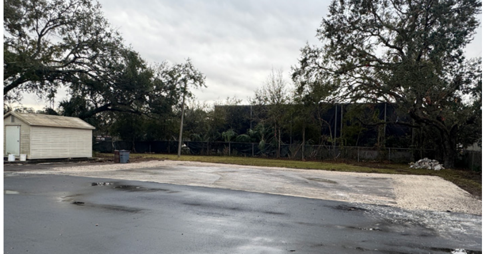
The area where the wall stood was soft and unstable, so we had the area packed down with gravel. This will allow cars to drive to the back area for additional parking.
