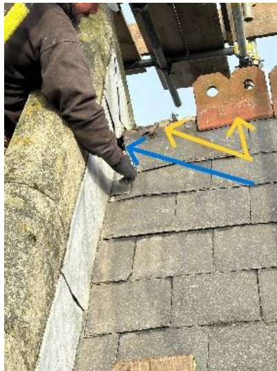
Photo 12 Missing lead flashing flashing.
