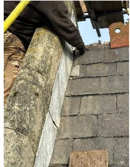
Photo 13 Apex Cresting not bedded in mortar
