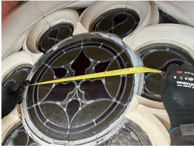
Photo 10 Circular Stained-Glass window found bowed inwards & at risk of failure
