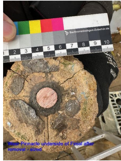
Photo 5 Underside of finial, extent of cracking to core clearly visible
