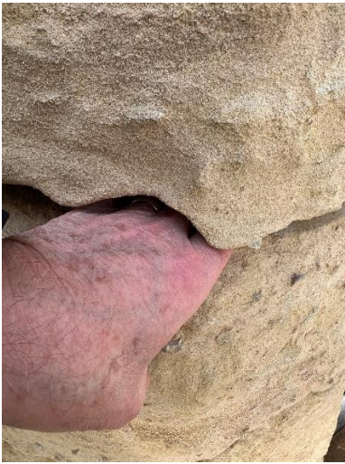
Photo 3 Extent of erosion at joints hand showing depth of weathering
