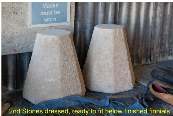
Photo 14 2 nd Stones ready to be installed
