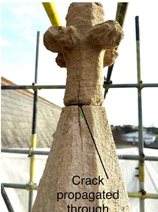
Photo1 – Top of west pinnacle the finial after cleaning, 3 cracks clearly visible.
