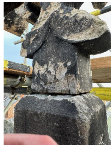
Photo 8 further detail of cracking
