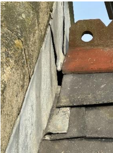
Photo 11 Apex of roof lead flashing incomplete
