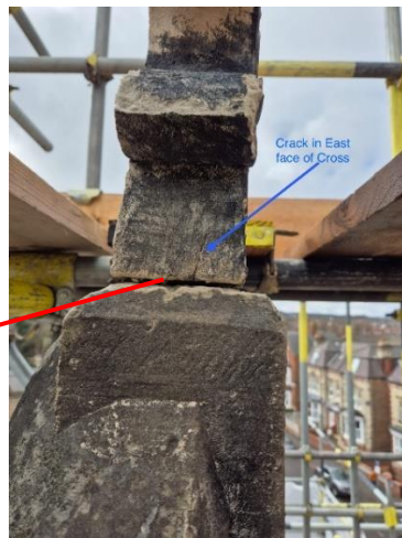
Photo 7 Detail of cracking in Cross base
