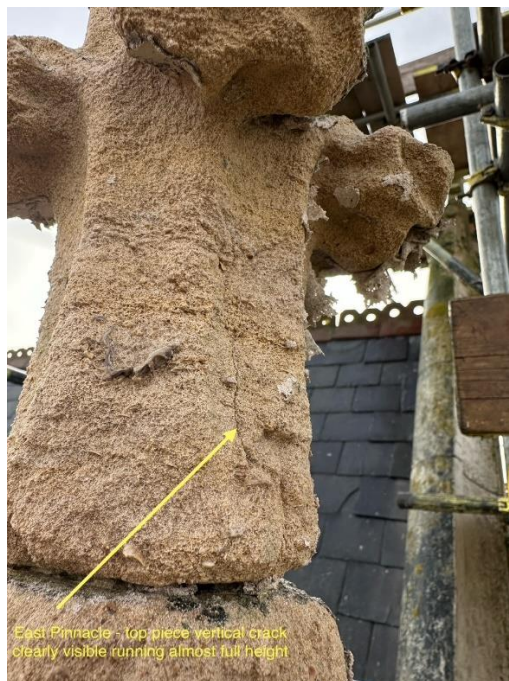
Photo 2 – East pinnacle finial showing similar cracking as west. NB Finial is top decorative part
