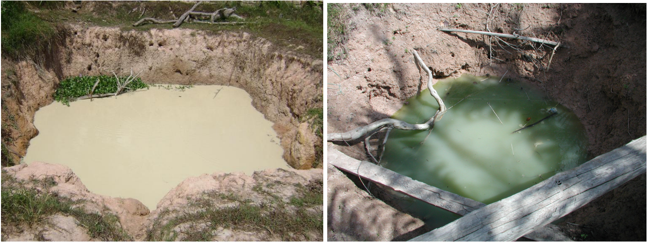
Typical traditional pit wells – used prior to receiving a pump well
