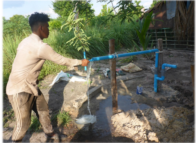
Life with a PVC pull pump well
