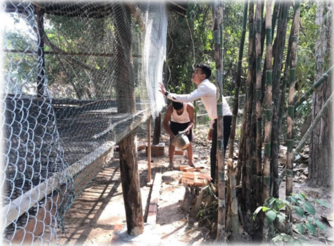
Building the chicken barn >
