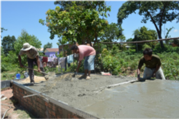
Construction of the filtration/hand washing station
