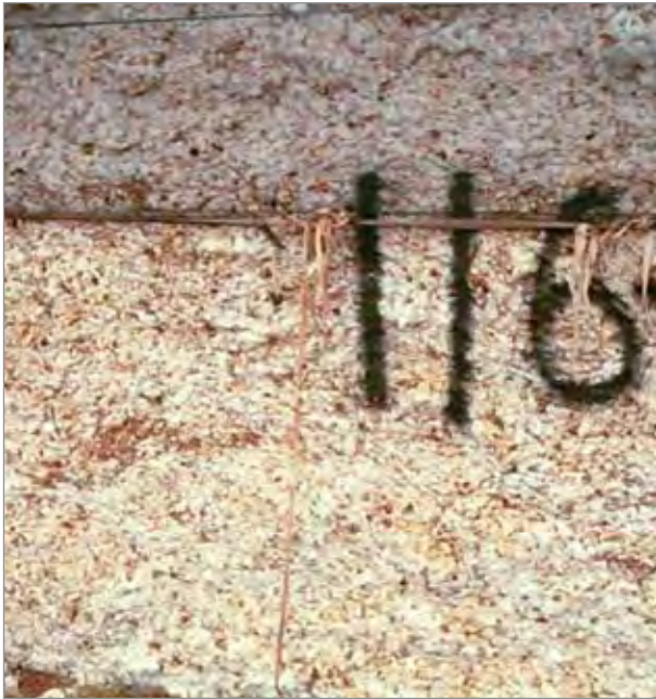
Figure 20 Baling twine and other plastic materials should not be used as tie-downs. Module tape can be used to hold down covers in high wind regions. The tape should be placed under the module before it is formed, and not through the module. (Photo by Alan Brashears.)
