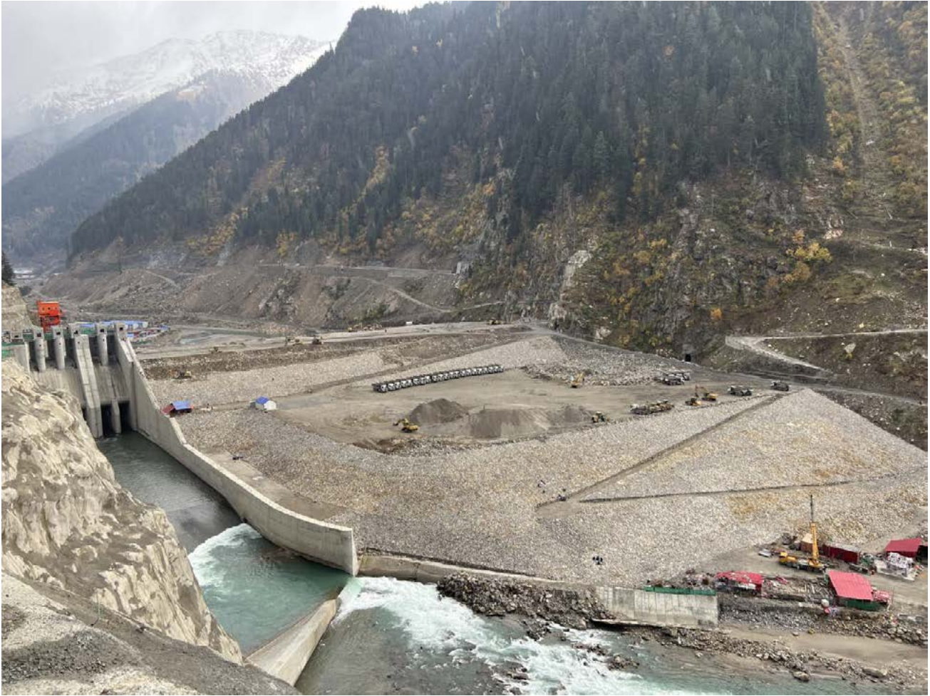
Photo 3 Rockfill dam under construction
