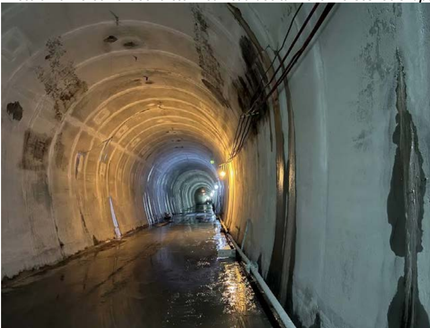
Photo 5 Reinforcement concrete lined headrace tunnel of horseshoe shape
