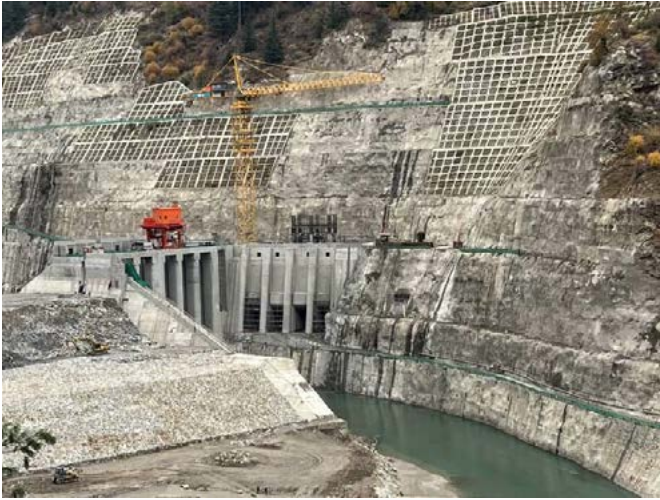
Photo 4 Spillway and power intake under construction
