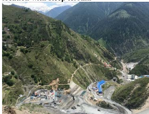
Photo 2 Construction site at the powerhouse location with steep terrain
