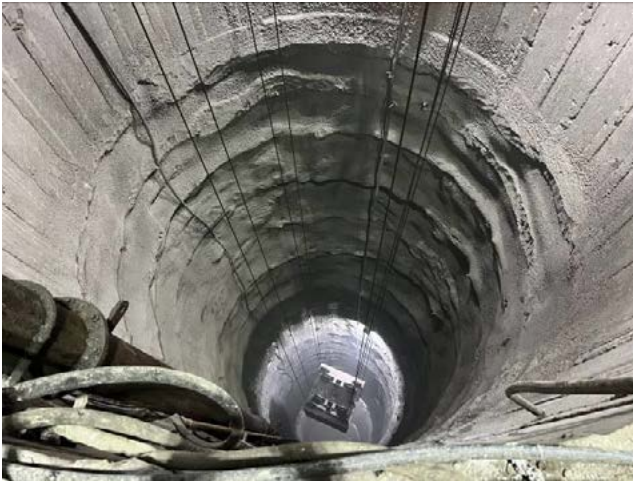
Photo 6 Power shaft under construction
