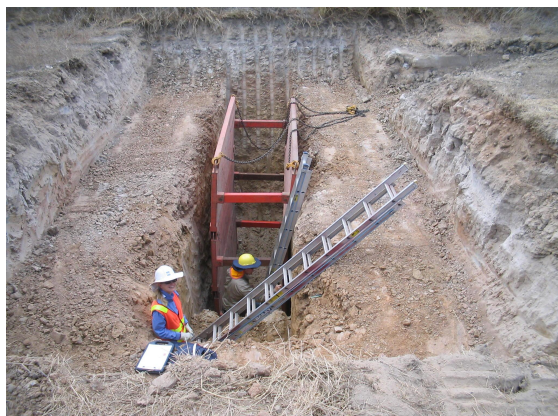
Figure 16 Shored pit used to provide access for fissure mapping.
