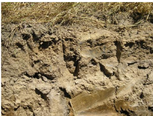
Figure 8 Type A Fissure
