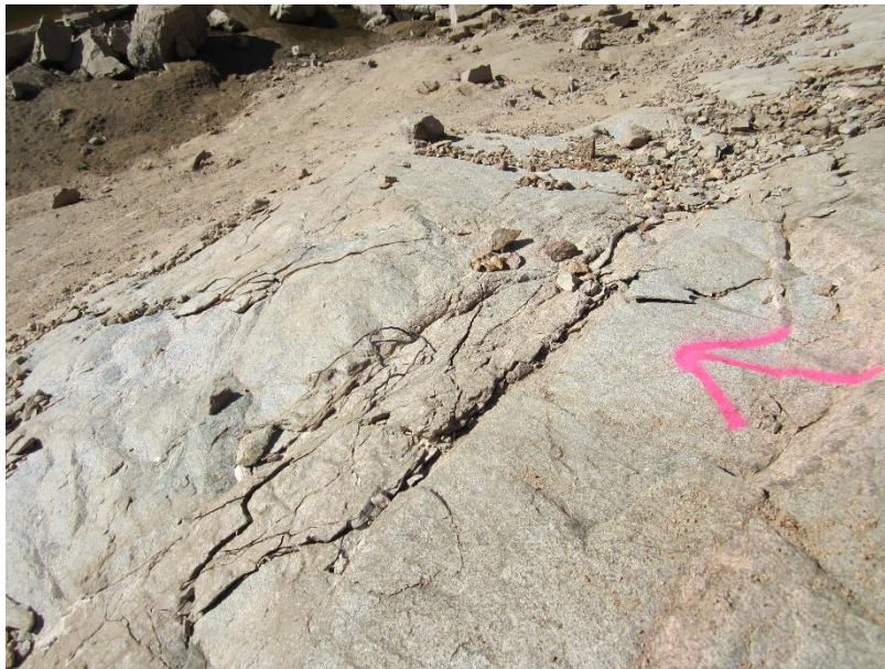
Figure 2 Indication of highly stressed rock mass at a dam in Queensland.
