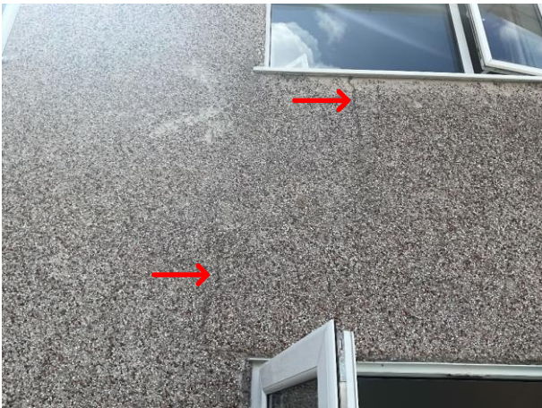
Additional views of cracks to rear elevation render.
