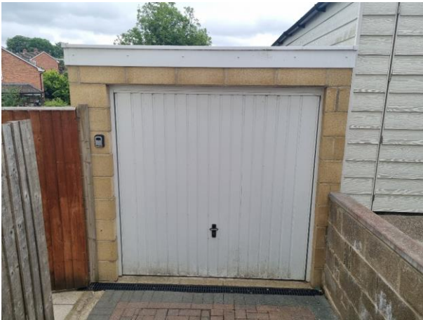
General view of garage.
