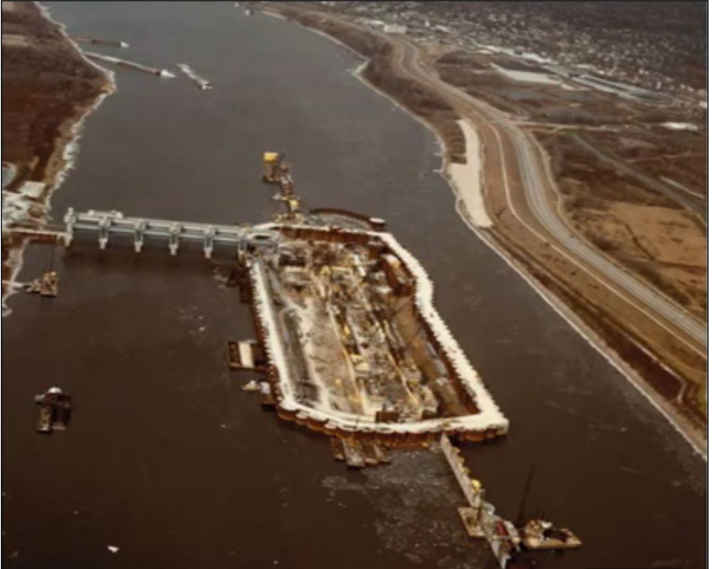
Figure 4-1 Melvin Price L&D Construction Photograph
