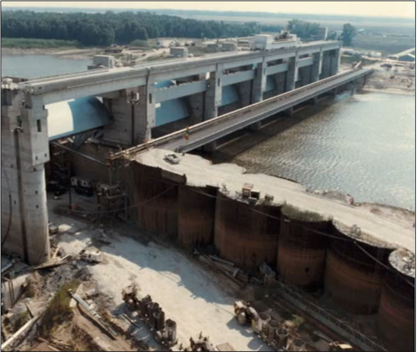
Figure 4-2 Melvin Price L&D Construction Photograph
