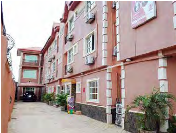
HardRock Hotel and Suite, Lagos
