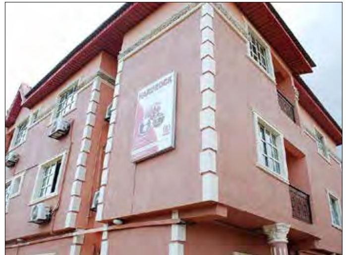
HardRock Hotel and Suite, Lagos
