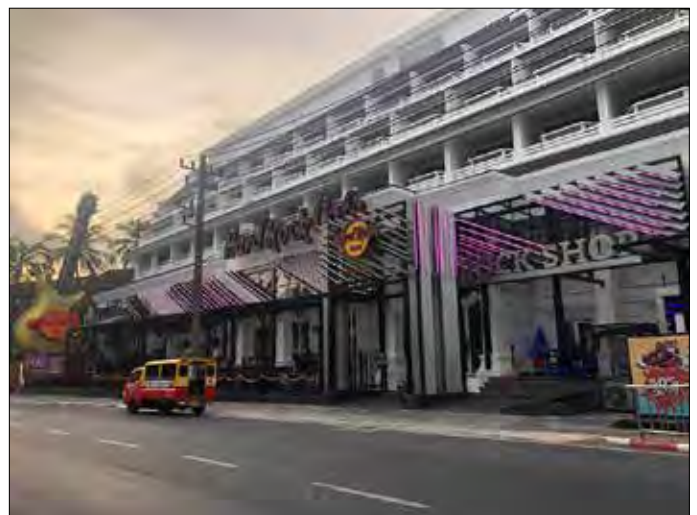
Phuket (new facade)
