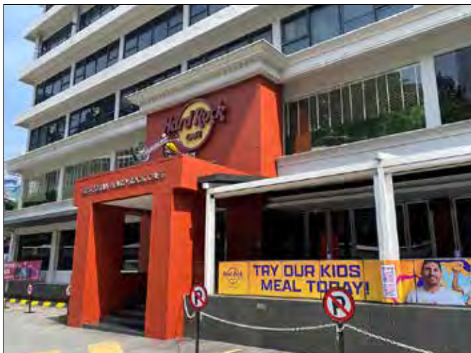
Kuala Lumpur (new facade)
