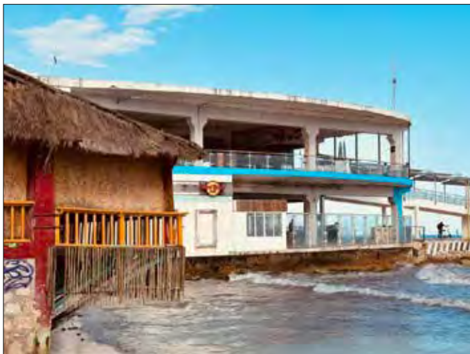
Playa de Carman Ferry Terminal (closed December 2023)
