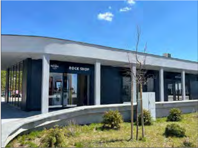
Kotor Cable Car Photo by Achim Sujer
