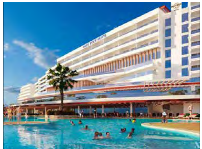
Fortaleza (under construction)
