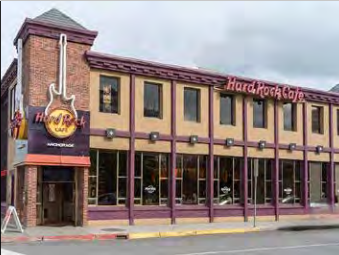
Anchorage (side view) (closed March 2020)
