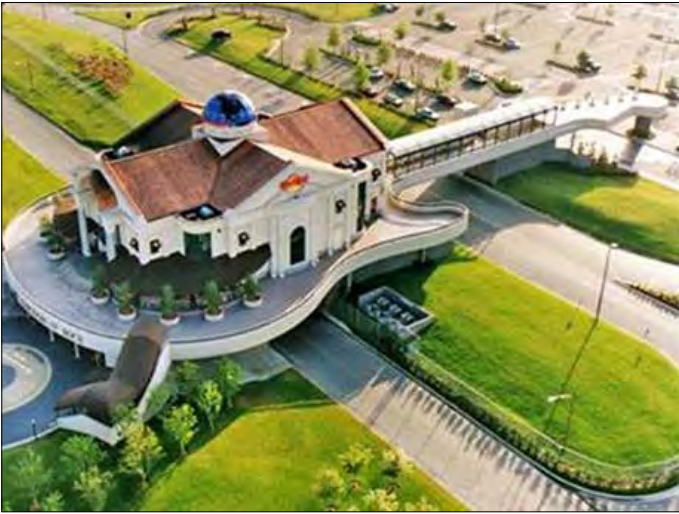
Orlando at Universal Studios (old location, closed December, 1998)
