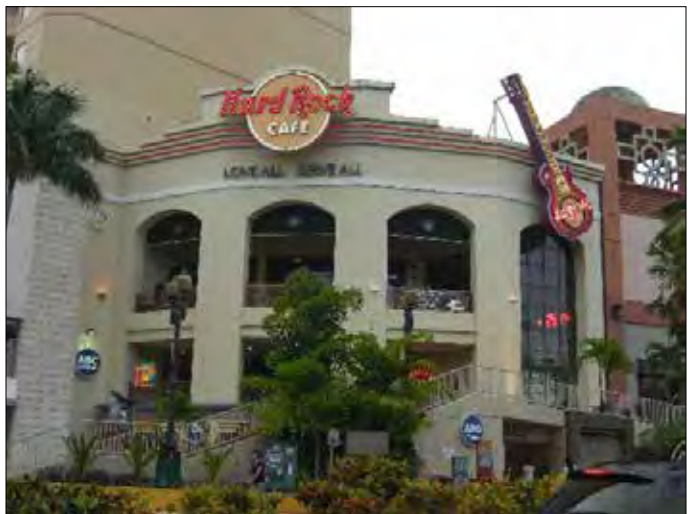
Guam (new facade, guitar replaced car, smaller building)
