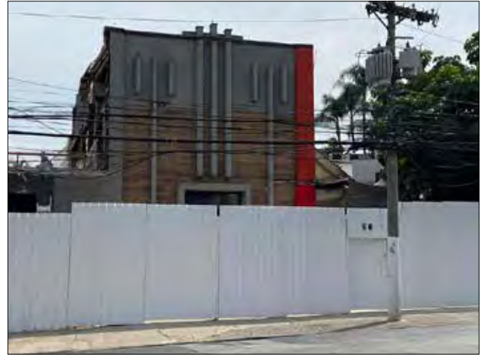
Sao Paulo (under construction)
