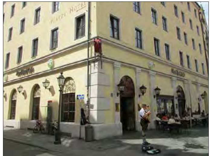
Munich (new facade)
