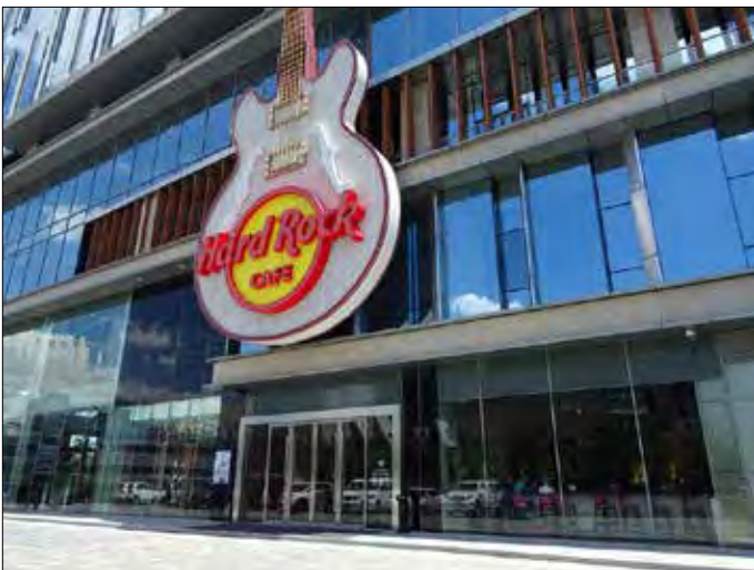
Shenzhen at the Hard Rock Hotel (entrance)
