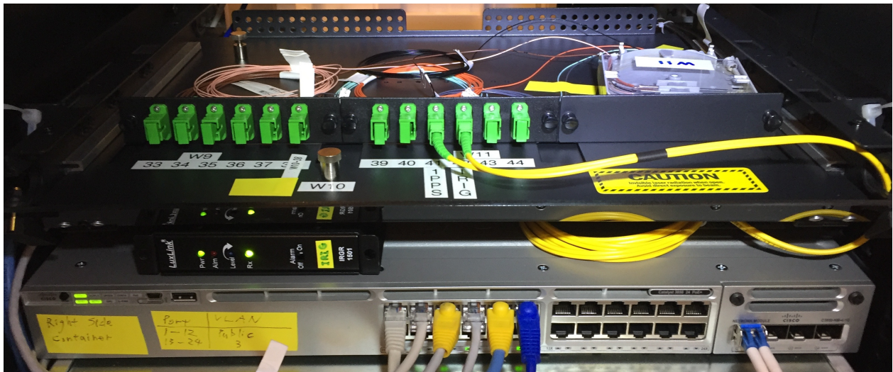
Figure 3 – Right Side Container splice chassis for W9 and W10 from control room, and W11 from maser house.
