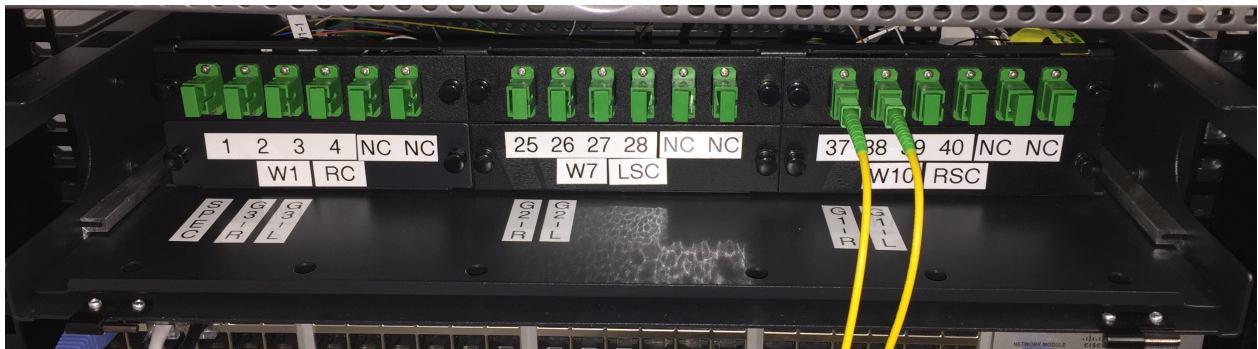
Figure 4 - Control trailer splice chassis for W1 to Rx cabin, W7 to Left Side Container, and W10 to Right Side Container.
