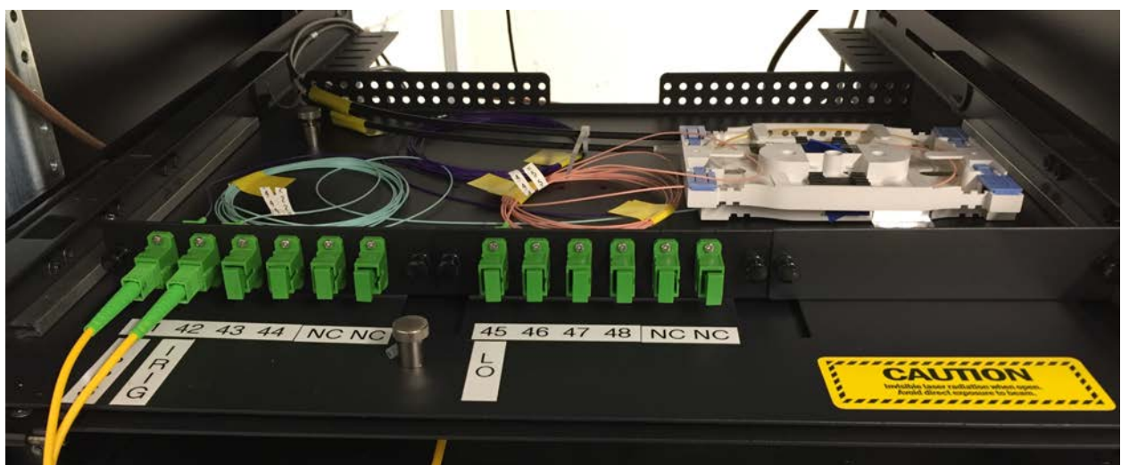
Figure 2. Maser house splice chassis for W11 to RSC and W12 to Rx Cabin
