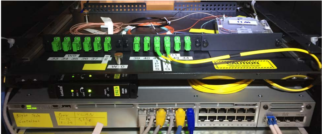
Figure 3. RSC splice chassis for W9 and W10 from control room, and W11 from maser house
