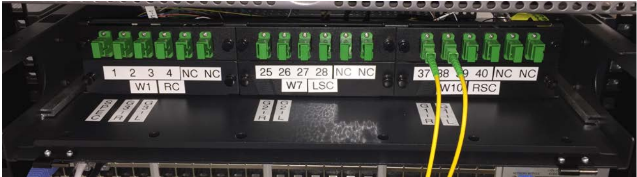
Figure 4. Control container splice chassis for W1 to Rx cabin, W7 to LSC, and W10 to RSC
