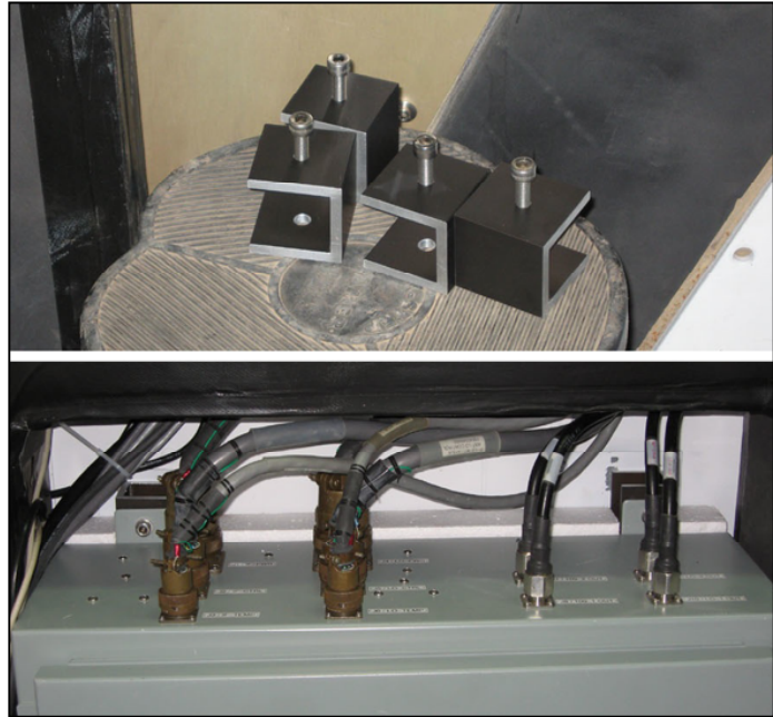
Figure 3 2-inch aluminum spacers (top), antenna 6 with spacers and foam insulation (bottom).
