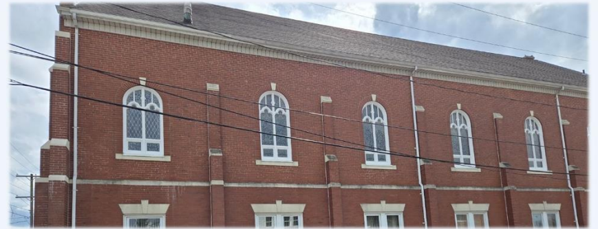
HOLY CROSS CHURCH WINDOW RENOVATIONS COMPLETED! MARCH 2025
