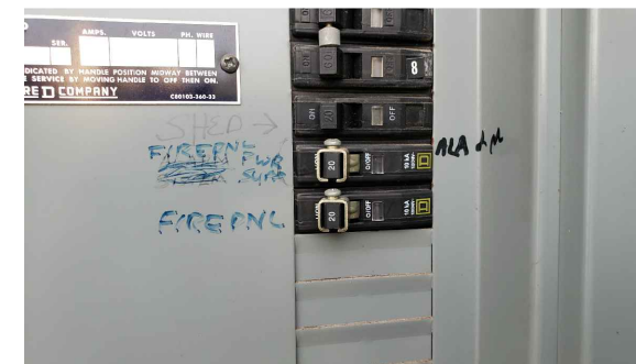
BUILDING B F.A. CIRCUITS
