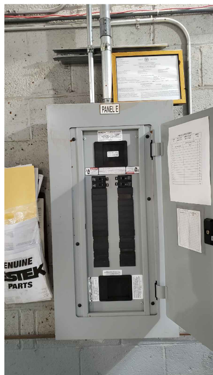
BUILDING C PANEL E
