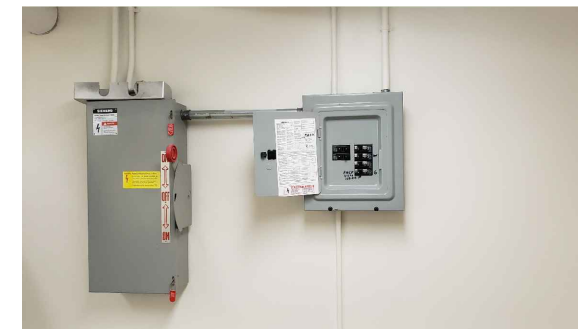
BUILDING C F.A. PANEL & DISCONNECT
