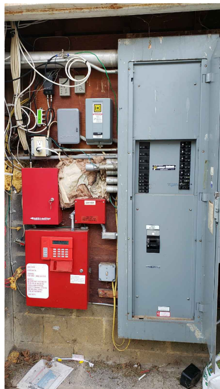
BUILDING A SERVICE CLOSET
