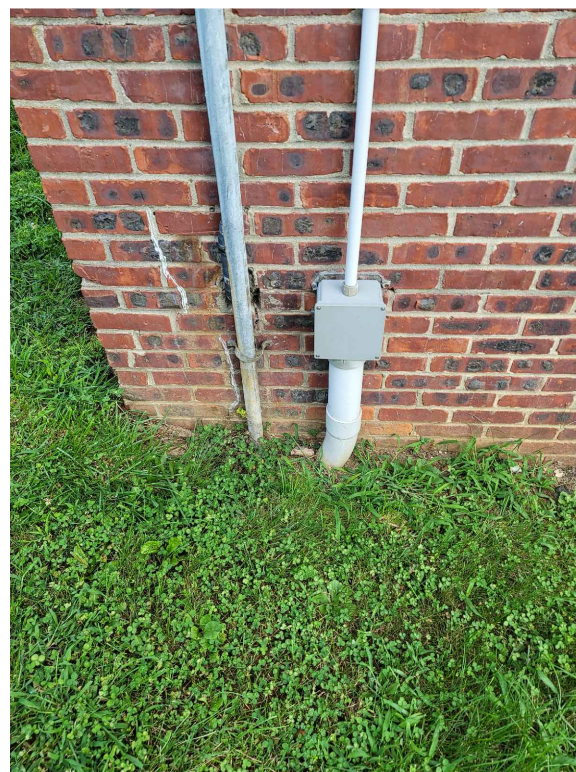
EXIST. UNDRGRND. CONDUIT BLDG C
