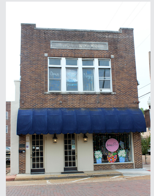
The original first floor storefront of these buildings has been removed and inappropriately replaced with incompatible materials and entry configurations.
