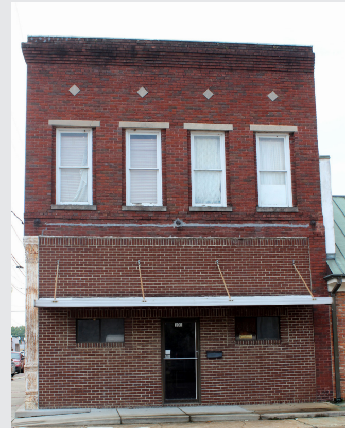
The original first floor storefront of these buildings has been removed and inappropriately replaced with incompatible materials and entry configurations.
