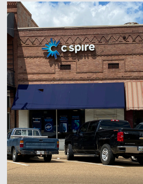
Inappropriate channel letter sign.
