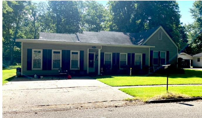
Inappropriate addition on the front of a house.
