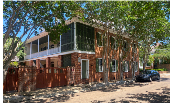
Appropriate addition on a rear porch enclosed with faux shutters.
