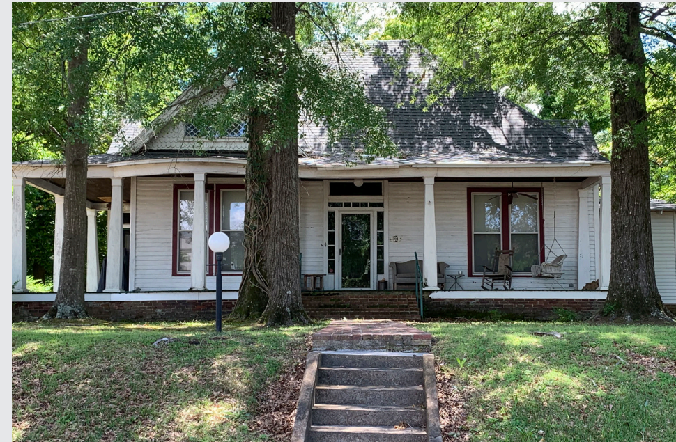
Original historic porch in downtown Water Valley.
