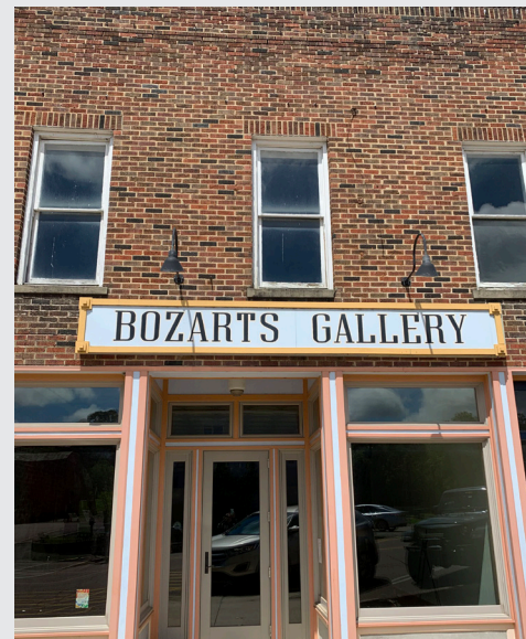
Appropriate signage lighting.
