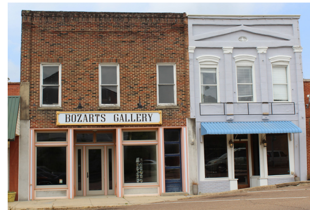
Historic brick was traditional unpainted, while historic stucco and woodwork were traditionally painted.
