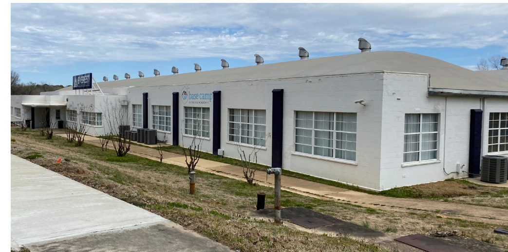
The Everest Building is an industrial building featuring large metal windows with awning sections that swing outward.
