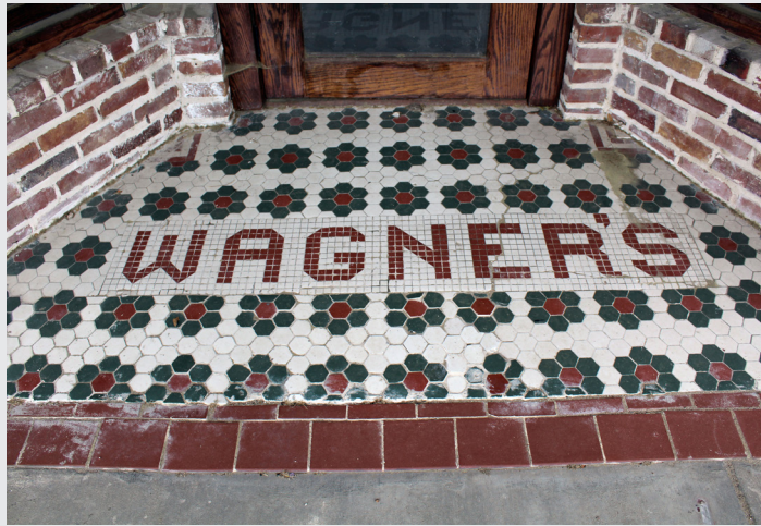
Original tiled entryway.
