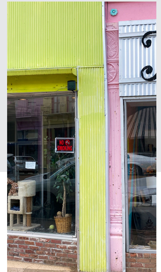
This original metal pilaster has been covered by metal paneling on the adjacent building.
