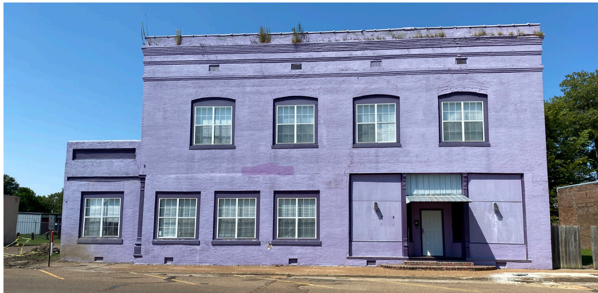
The original windows on this building have been replaced with windows of inappropriate size, shape and material. The openings have been filled around the replacement windows. The original entry door has also been replaced and infilled.
