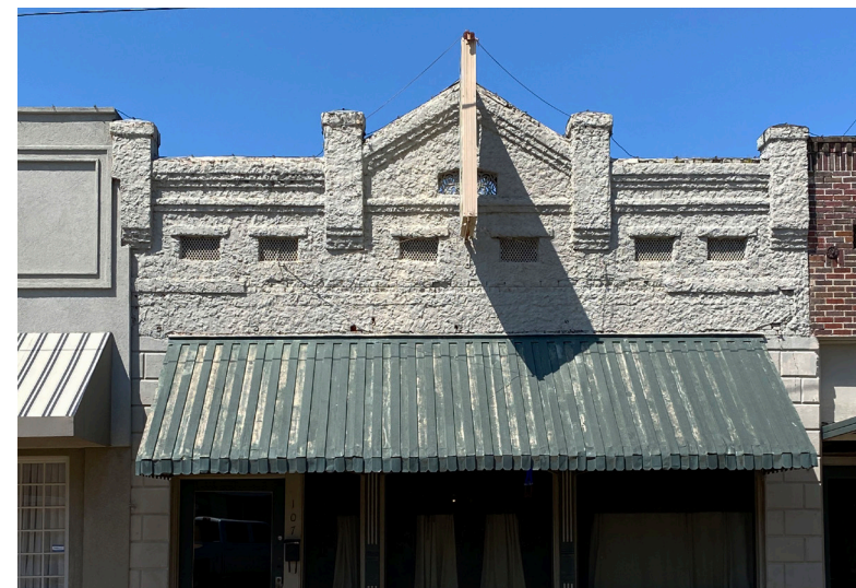
The original façade material has been covered by textured stucco.
