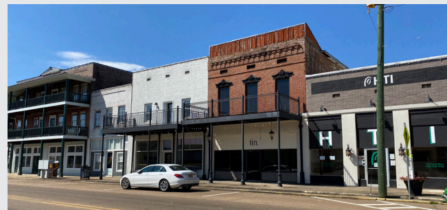
Two and three story storefront block.
