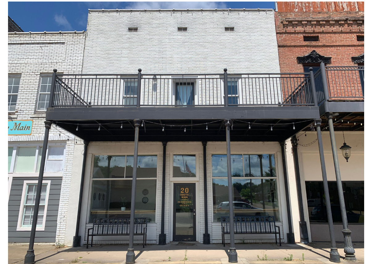
Appropriate wood full-lite entry door in the historic district.
