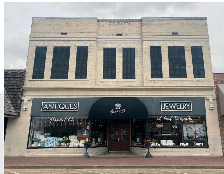
The original windows on this building have been replaced with windows of inappropriate size, shape and material. The openings have been filled around the replacement windows. The original entry door has also been replaced and infilled.
