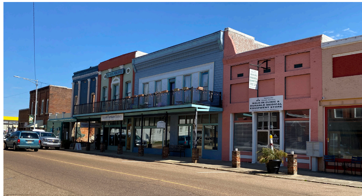
Commercial roof lines in Water Valley.
