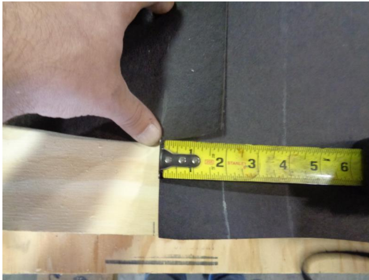
Photo No. 15 Assembly #2 2-inch Overlap
