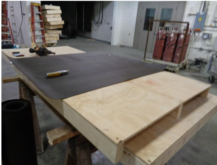
Photo No. 1 Assembly #1 Deck Construction (Typical)
