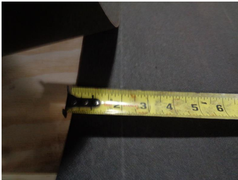
Photo No. 2 Assembly #1 2-inch Overlap (Typical)
