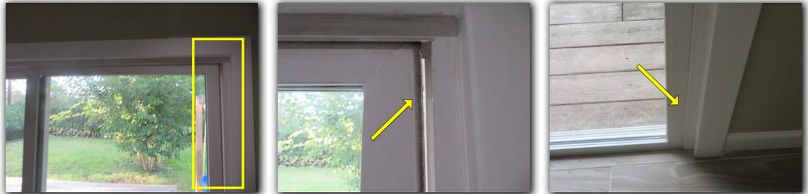
The latch bolt on the door lock is not latching in the strike plate in Backyard Door. Door hardware should be repaired and/or replaced as needed for proper operation of door and safety reasons.
