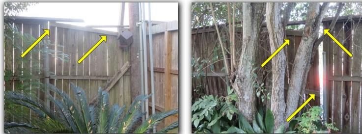
The gate on the fence was observed to have a broken latch. This can be repaired and/or replaced as needed.
