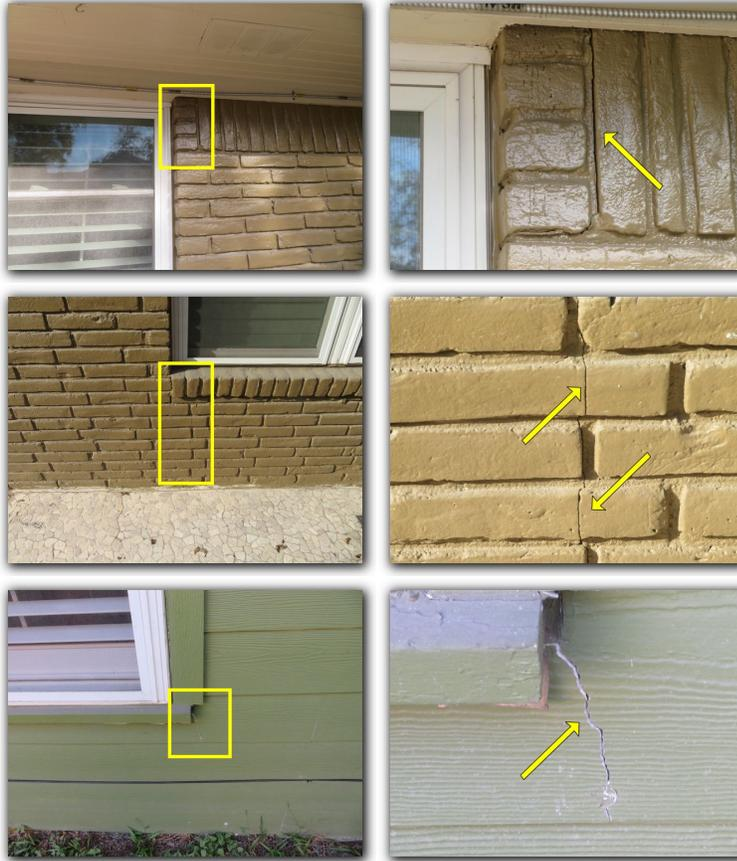
Typical cracks were observed on the walls of multiple rooms.
