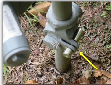
Sediment trap was observed to be not installed in the gas supply piping. The sediment trap serves as a collection chamber for sediment and moisture to reduce the risk of clogged gas valve(s) or burner(s). This should be corrected by a qualified professional for proper operation of the heating unit.
