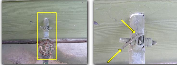
Only one grounding rod (grounding electrode ) was observed on the property. Current building standards require installation of two grounding electrodes. The presence of a proper grounding electrode system should be verified or a proper grounding electrode system should be installed for safety. **This house predates the adoption of this standard; however, this should be corrected for safety reasons.**
