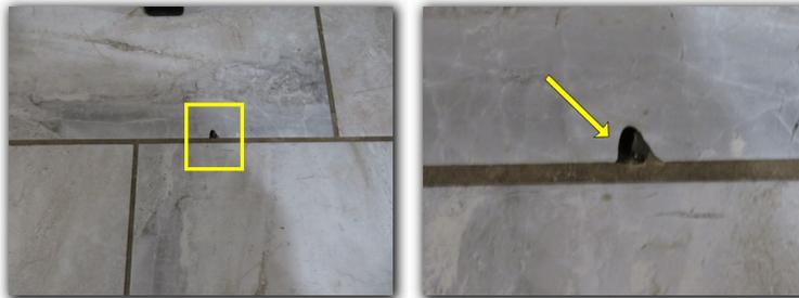
Cracks were observed on the tile floor in the Foyer.
