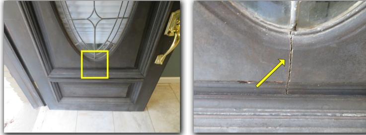
Multiple doors were observed to be out-of-square. This may be an indication of structural movement, sub-standard installation or door hardware issues.
