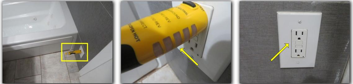
Tamper resistant receptacles were observed to be missing on the property. Current electrical standards require tamper resistant receptacles in new and renovated homes because it is the most effective way to prevent injuries associated with electrical receptacles, especially to children. **This property predates the adoption of this standard; however, this should be corrected for safety reasons.**
