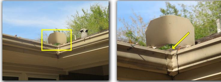
Nails were observed to be under driven on the gutter on the right side of the property. The nails should be fully driven to secure the gutter to the eave.
