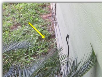
*Notes:* Grading and drainage is visually inspected for adverse conditions at the area adjacent to the foundation. It is recommended to maintain positive drainage away from the foundation for minimum of 6 to 10 feet and keep 6 to 8 inches of slab exposed.
