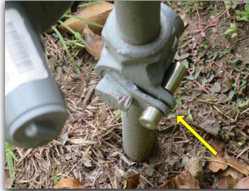
Sediment trap was observed to be not installed in the gas supply piping. The sediment trap serves as a collection chamber for sediment and moisture to reduce the risk of clogged gas valve(s) or burner(s). This should be corrected by a qualified professional for proper operation of the water heater.
