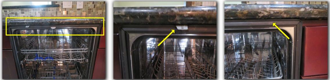
The dishwasher lacks an air gap device or a high loop. Air gaps are now standard equipment to assure a separation between supply and waste water. It is advised that one be installed or the waste pipe properly configured to prevent back flow of waste water into the dishwasher.
