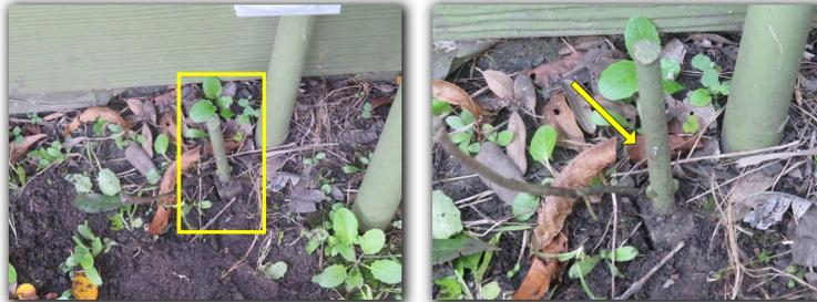
The grounding conductor was not connected to the grounding rod on the right side of the property. The purpose of this grounding rod should be evaluated by a qualified professional.
