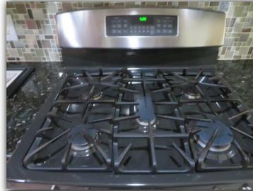
The cooking range was not secured to the wall or cabinet. An anti-tip bracket should be installed for safety reasons to avoid the cooking range from tipping over and causing injury.
