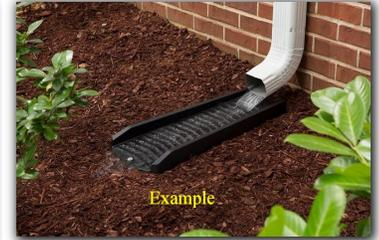
Areas of neutral and/or negative drainage that will route runoff from rain toward the foundation were observed on the property. The grading can be improved and/or French Drain installed to promote the flow of storm water away from the house. The ground should slope away from the house a minimum of 6 inches within the first 10 feet or to a swale if 10 feet is not available.
