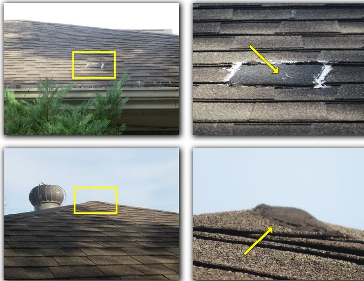
Damaged roof shingles were observed at multiple areas of the roof. Damaged and/or missing roofing material should be repaired to reduce the risk of water intrusion.
