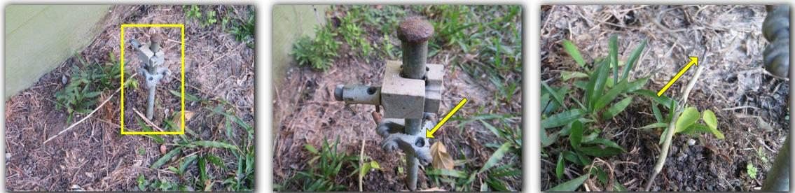
A disconnect containing fuses was observed next to the electric meter. The purpose and safety of this disconnect should be evaluated by a qualified professional.
