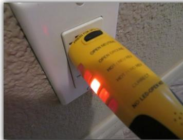
Several outlets were observed to have open ground in the Drawing Room. These outlets and the circuits should be evaluated and corrected by a qualified professional for safety reasons.
