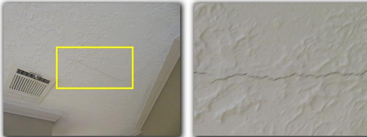
Evidence of prior repairs was observed on the ceiling of the Hallway, and, Bedroom 3.
