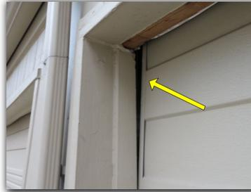
The roll-up garage door frame was observed to have a sag and separation.
