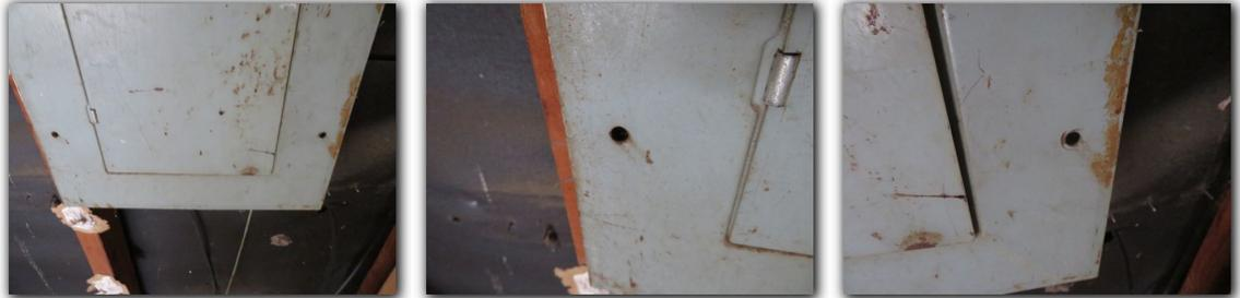
The electrical panel screws were observed to be replaced with sharp pointed sheet metal screws. These screws are unsafe and can pierce and/or damage the panel wiring. These should be replaced for safety reasons.
