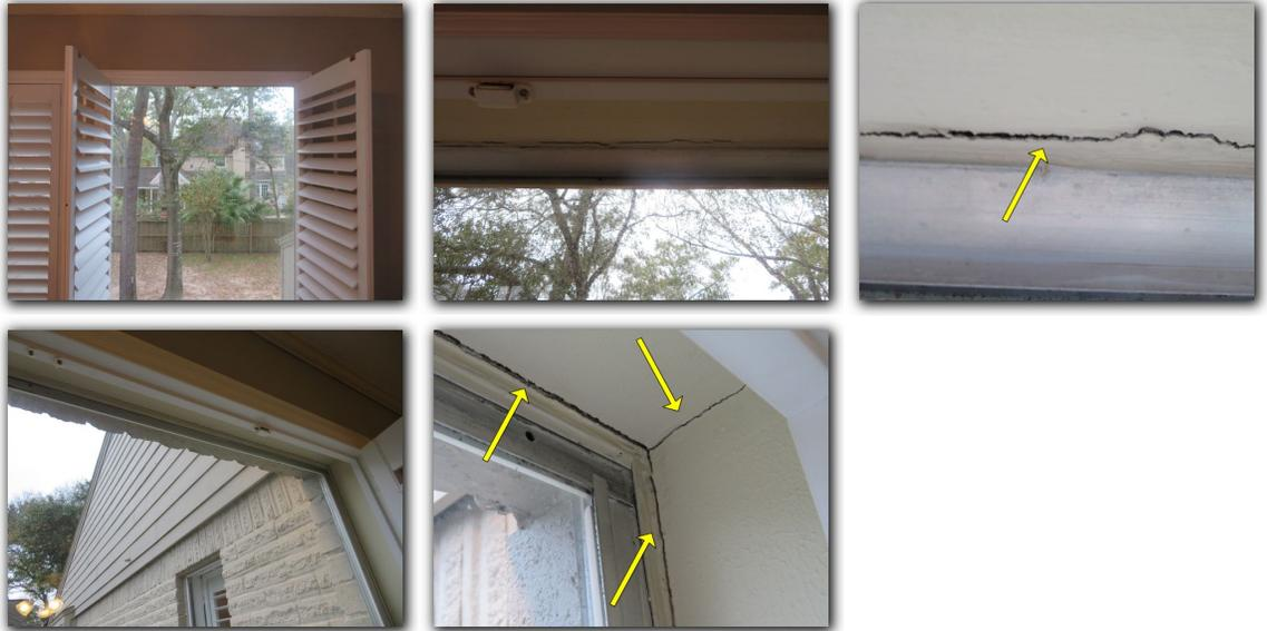
A window did not latch when closed in Bedroom 2. The window hardware should be adjusted for safety reasons and proper operation of the window.
