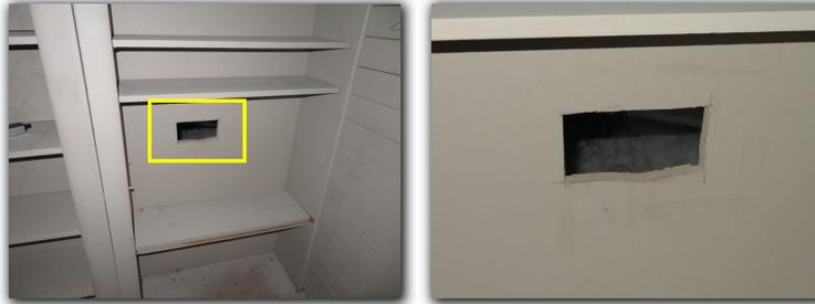
The attic access doors were observed to be not insulated. It can be weather stripped and/or insulation installed to increase the efficiency of the heating or cooling system.
