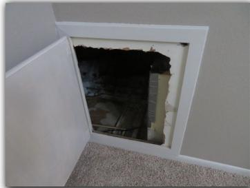
Insulation was observed to be Up to 4 inches thick on the attic floor. Current building standards recommend 13 - 14 inches insulation thickness for most southern climates. This can be improved or additional insulation can be installed as needed.
