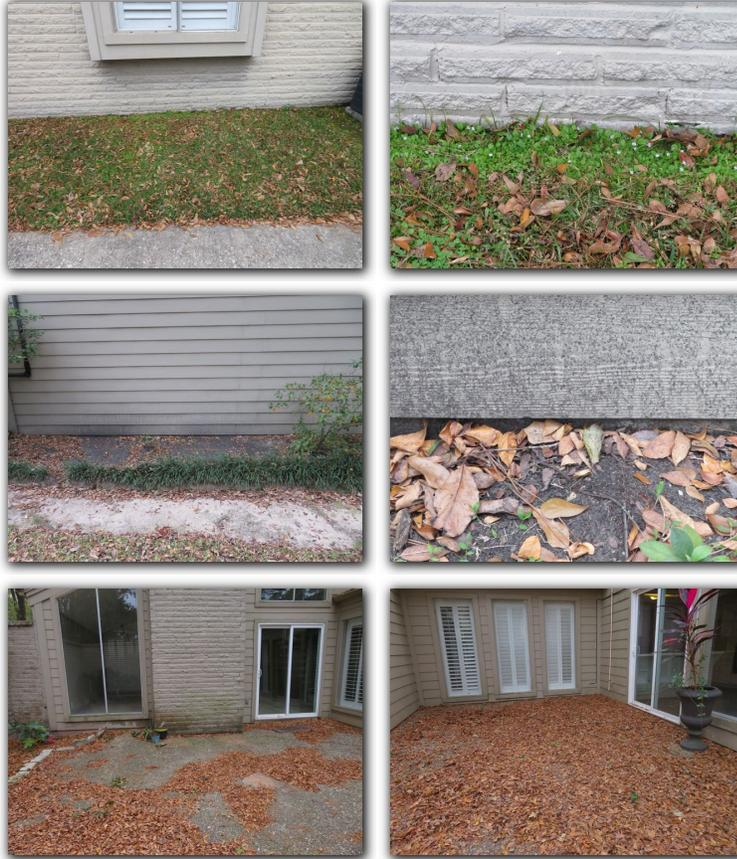
Roots from trees were observed near the foundation and may cause foundation damage as the tree grows and the root system expands. Monitor all areas of the foundation in close proximity to the trees for signs of damage. If signs of damage appear (such as cracks), the tree and/or the roots may need to be removed. The potential for damage from tree roots varies with tree species.
