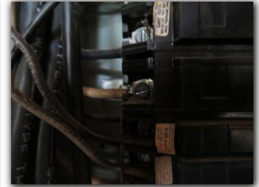
Neutral and Ground wires were observed to be double tapped under one lug. Current electrical standards require that neutral wires cannot be double tapped and a neutral and a ground wire cannot share one lug. This should be corrected for safety reasons.
