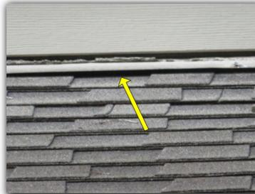
The valley flashing was observed to be loose. It should be secured and sealed to reduce the risk of water intrusion. All exposed flashing and roof penetrations should be examined and sealed as necessary.
