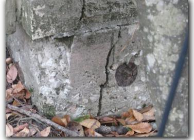
Spalling was observed on the foundation beam.
