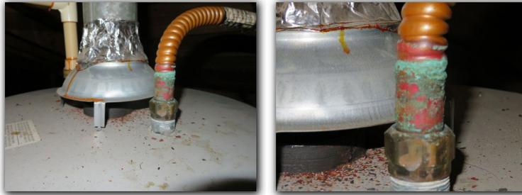
Foil was observed to be wrapped around the water heater vent flue. This is not an approved and recommended method of installation and repair.
