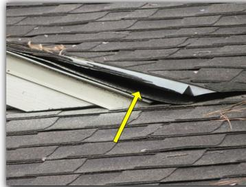
The vent flashing was observed to be loose and should be secured to reduce the risk of water intrusion.
