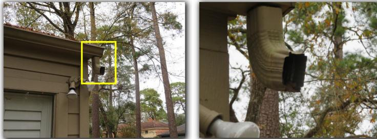
Splash blocks were observed to be missing under multiple downspouts. Splash blocks can be added to prevent soil erosion and for proper drainage of rain water. Rain water should flow away from the structure at the points of discharge, at least 3 feet away from the foundation.
