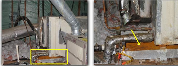
Damaged and/or missing insulation on the refrigerant line was observed at the evaporator coil unit in the attic. The cold copper tubing in contact with warm humid air causes moisture in the air to condense and then drip off of the refrigerant line. This should be repaired and/or replaced to reduce the risk of moisture intrusion.
