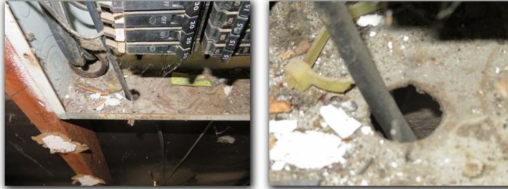
Gas and water pipes on the property were observed to be not bonded to the electrical system. Current building standards require that the gas and water pipes should be bonded to electrical system. This condition should be corrected by a qualified professional for safety reasons.
