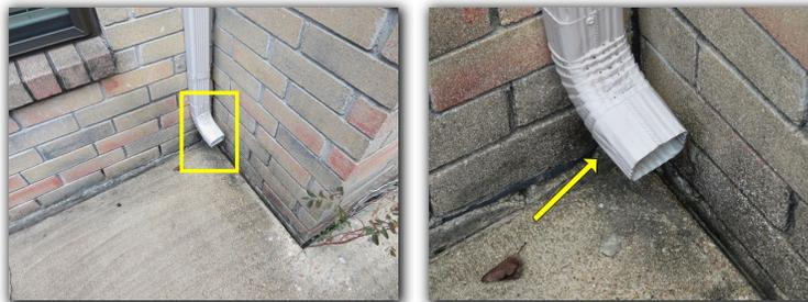
*Notes:* Grading and drainage is visually inspected for adverse conditions at the area adjacent to the foundation. It is recommended to maintain positive drainage away from the foundation for minimum of 6 to 10 feet and keep 6 to 8 inches of slab exposed.
