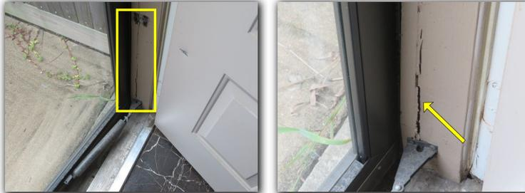
The front door was observed to be misaligned and hits/rubs the floor when opened/closed. This should be improved for proper operation of the door.
