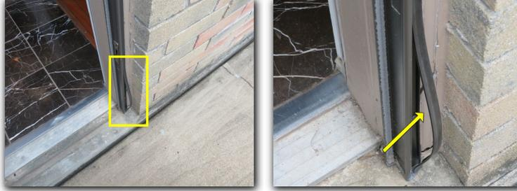
The door frame was observed to be cracked in the door frame of Front Door. This should be repaired to prevent further damage to the frame.
