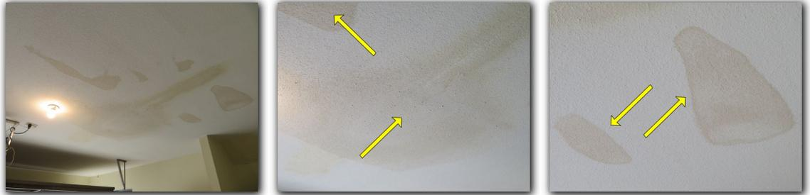
Typical ceiling cracks were observed in the Garage. This condition is very common and is not a structural concern.
