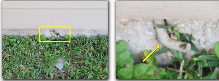
A drain pipe was observed to be exposed on the left side of the property and is not a structural concern.
