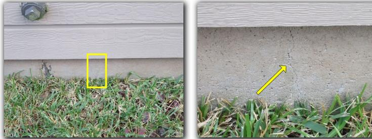
Evidence of parging was observed on the foundation perimeter beam on the right side, and, left back corner of the property. Parging is essentially a decorative mortar coat that is applied to the above grade foundation to act as a finish coat to hide surface imperfections, cracks, spalling, etc. Parging can be applied to new or existing foundation.
