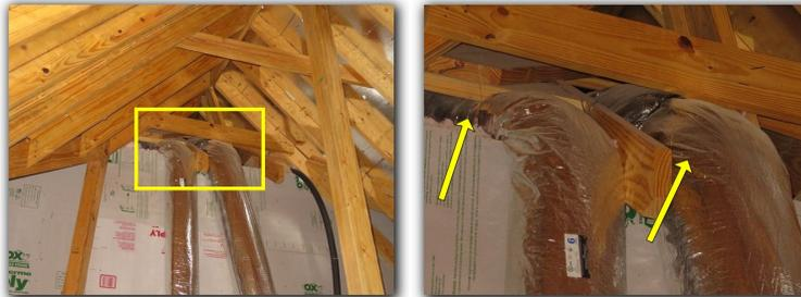
No heating or cooling was observed in the Master Bedroom, Master Bathroom and surrounding area when tested. The HVAC system and/or the duct system should be further evaluated and corrected by a qualified HVAC professional for comfort reasons.
