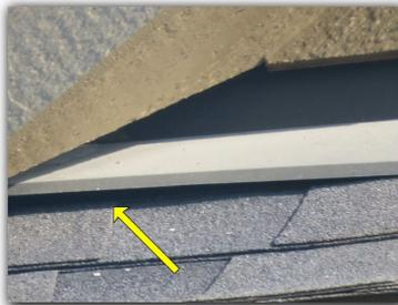
The wall flashing was observed to be loose on the front of the property. It should be secured and sealed to reduce the risk of water intrusion. All exposed flashing and roof penetrations should be examined and sealed as necessary.
