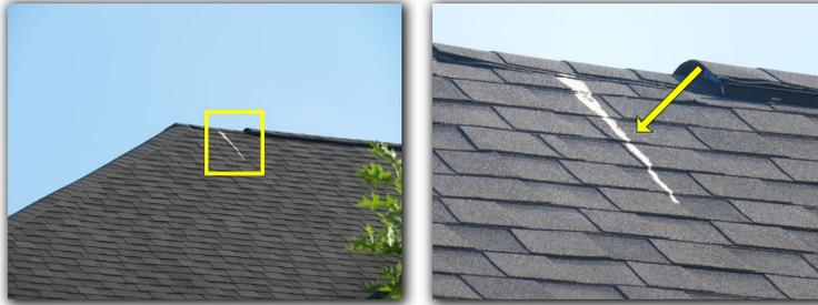
Damage was observed on the roof shingles on the front of the property. All damaged shingles should be repaired and/or replaced to reduce the risk of water intrusion.
