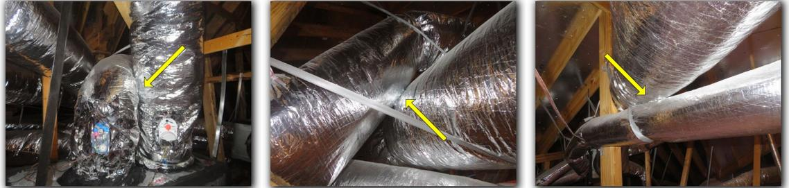
Supply air ducts were observed to be crimped between the framework and sheathing in the attic above the garage causing airflow obstruction. This should be corrected to improve the air flow.
