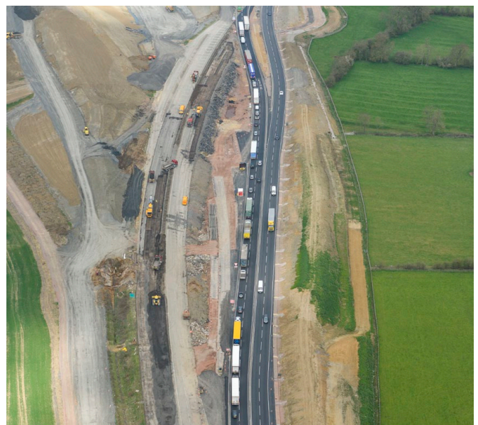
Both A14 eastbound and westbound traffic switched onto a temporary alignment to facilitate construction of the new A14-M6 westbound and A14-M1 northbound links.
