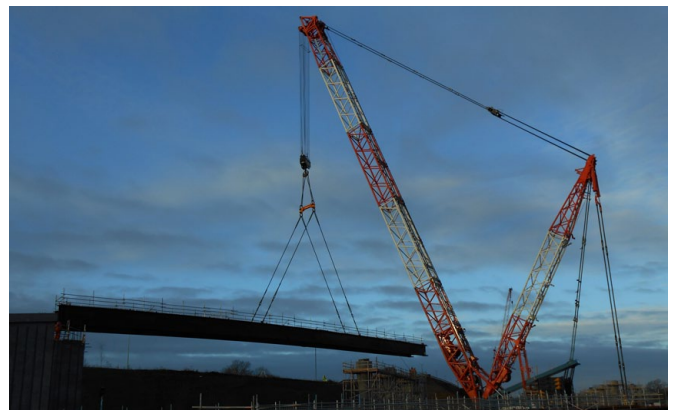
M6 to M1 bridge deck beams installed, and bridge deck works well under way. A 660 tonne crawler crane was used to lift the beams, with the heaviest lift weighing up to 200 tonnes.
