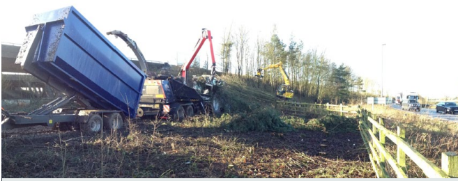
Vegetation clearance adjacent to the M1, M6 and A14 in January 2014 creates the space to build the eight temporary roads required to keep the junction 'open for business'.
