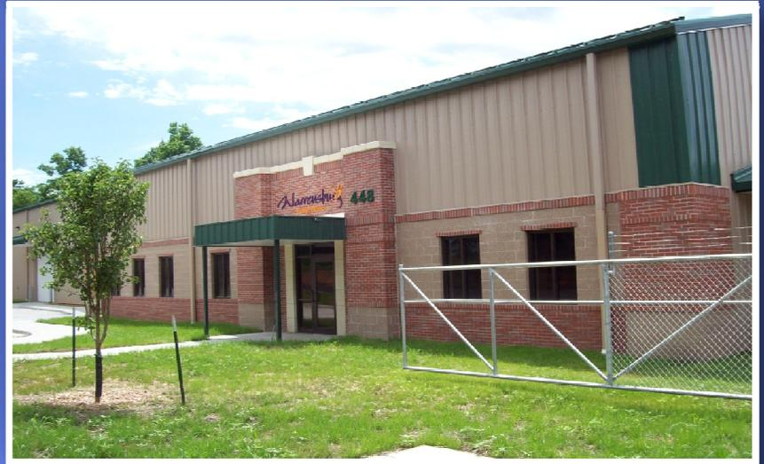
This project included the construction of a New Public Works building for the City of Warrensburg, Missouri. This building has an energy efficient design with all electric heat pump, extra building insulation, building "Tyvek" wrap and insulated glass windows.
