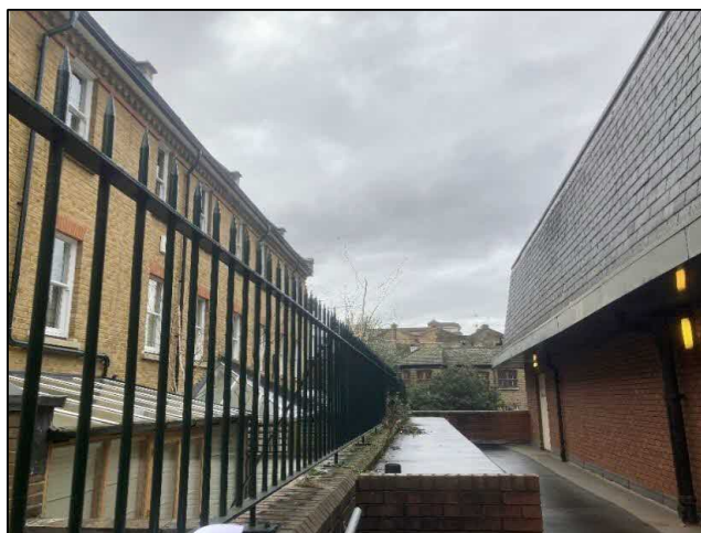
Photograph showing the rear of the houses at nos. 36-46 CIIP, looking onto the mansard roofs of M&S. Note the relative ground levels between the sites.
