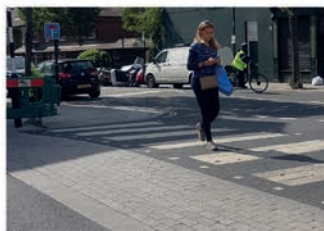
Raised table with granite ramps
