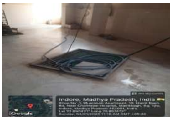
(i) Water Feature Inside Precinct
