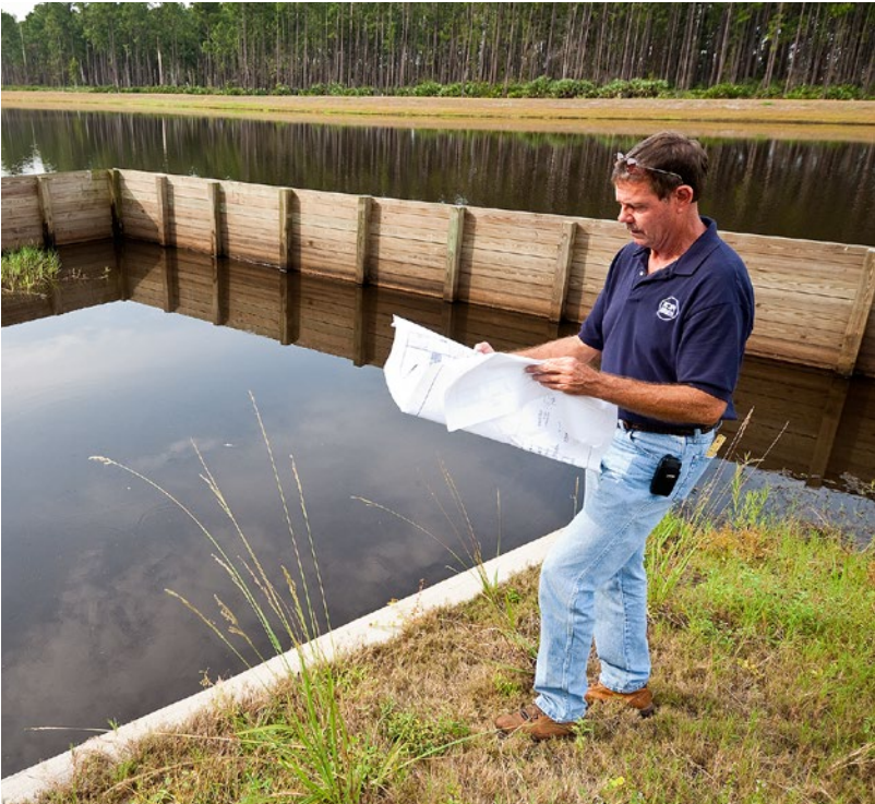
A District engineer inspects a stormwater system in St. Johns County.
