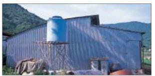
Livestock shelter is facing south so that the sun will gradually warm all parts of the structure. Air comes in from sides and goes out through the opening on top; triggering air circulation. Roof is made from galvanized steel sheet which further promotes air circulation
