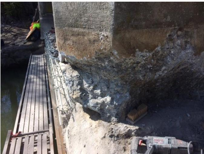
Deteriorated concrete under corroded steel on center pier
