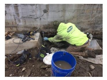
Deteriorated concrete under North Wall
