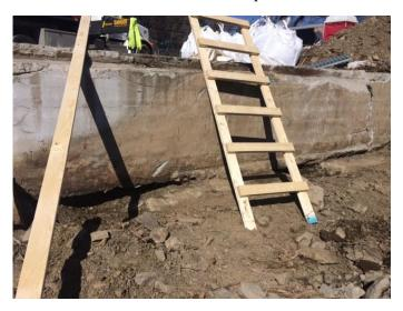
Deteriorated concrete under North Wall
