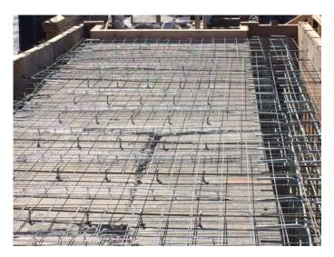
Steel Mesh installation on North Wall
