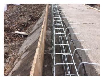
Steel rebar installation on North Wall
