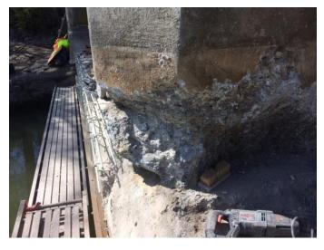
Deteriorated concrete under corroded steel on center pier
