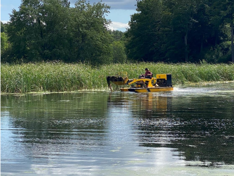
Figure 2: Hydroraking Activity in Section 6
