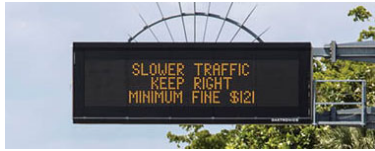
Overhead Dynamic Message Signs providing real-time travel information
