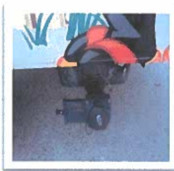
Liquid Waste Connection
