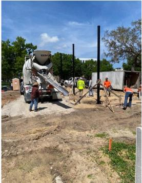
These photos show some of the work to dig the building footers, pouring the Jahna concrete by the TOMO Construction crew, and the completed pour of the footers giving a good idea of the footprint of the building.
