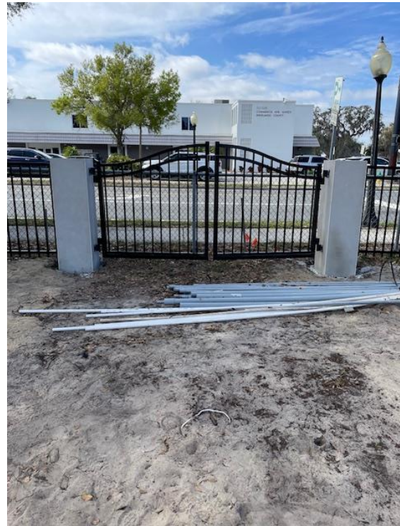
These photos show some of the aluminum fencing installed by the North American Fence Contractors Association, as well as some of the 29 columns after the stucco was applied. Later we will install caps on the tops of the columns. The gate is the "main" entrance on Commerce Street.
