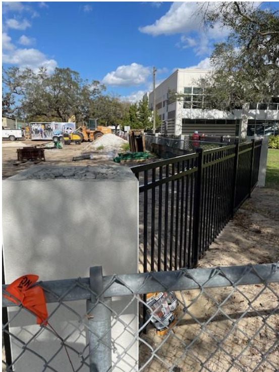
These photos show some of the aluminum fencing installed by the North American Fence Contractors Association, as well as some of the 29 columns after the stucco was applied. Later we will install caps on the tops of the columns. The gate is the "main" entrance on Commerce Street.
