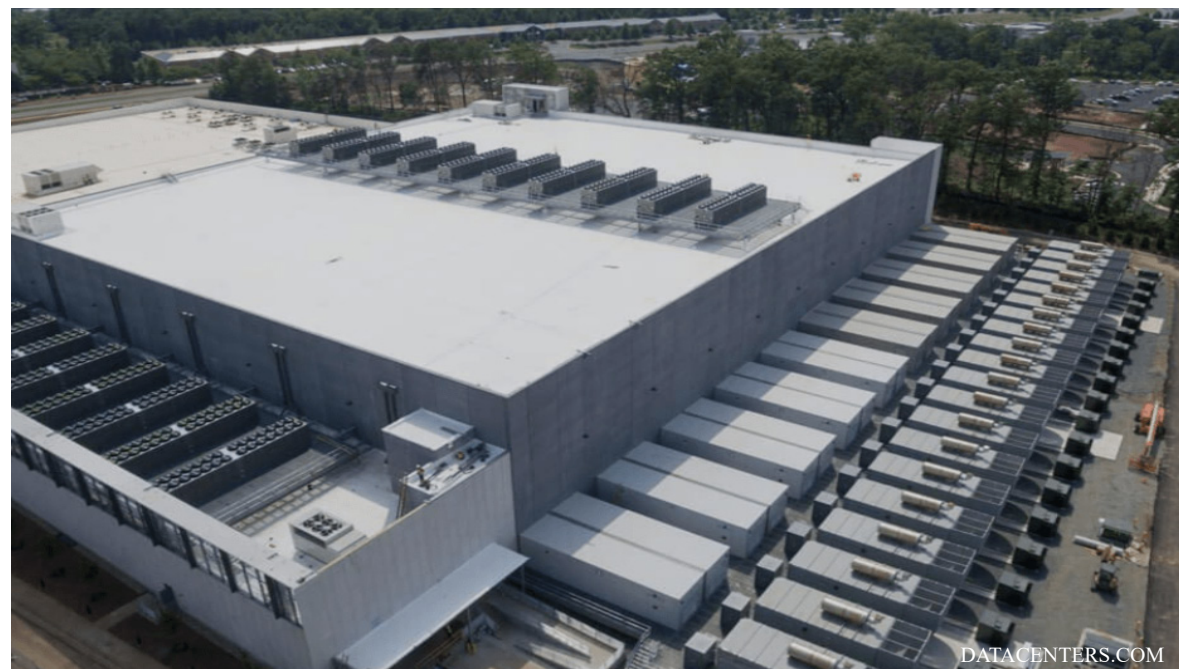
One of many data centers around Virginia.
