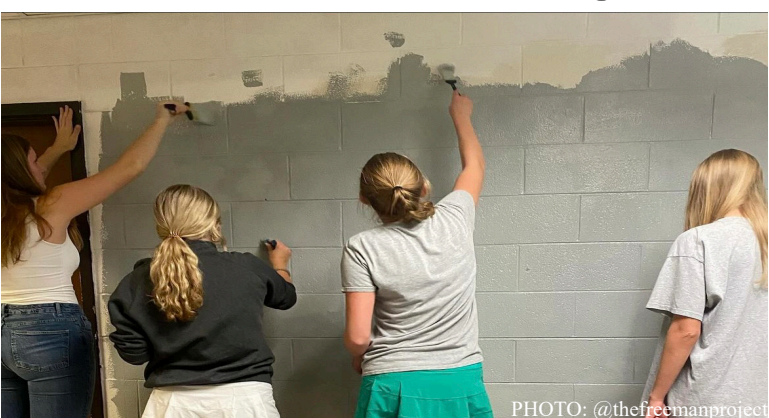
Freeman Project juniors work on painting the annex walls
