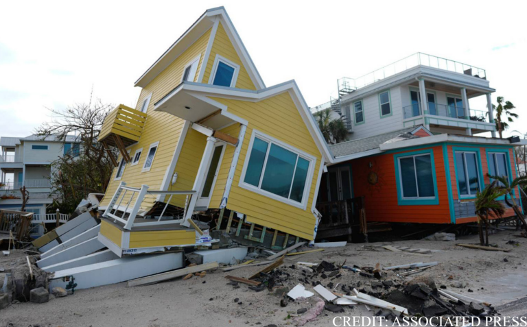
Destruction caused by Hurricane Milton in Florida
