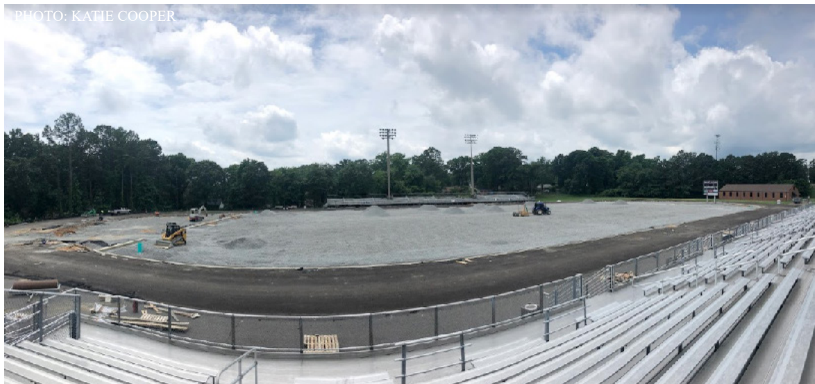
Panoramic view of the stadium field construction before turf is laid.
