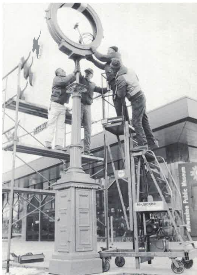
Placing the dial assembly on the column; from left: Steve Sanfilippo, Marv Rosenau, Joe Rebatzke, and Herb Smith.
