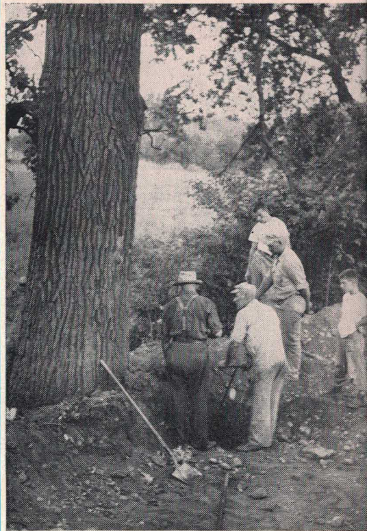
LAYING A DYNAMITE CHARGE
