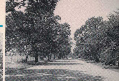
HIGHWAY 30 NEAR CROOKED LAKE, BEFORE WIDENING OPERATIONS.
