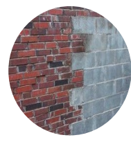
Exposed Existing Structure - Repurposed Concrete Block and Brick
